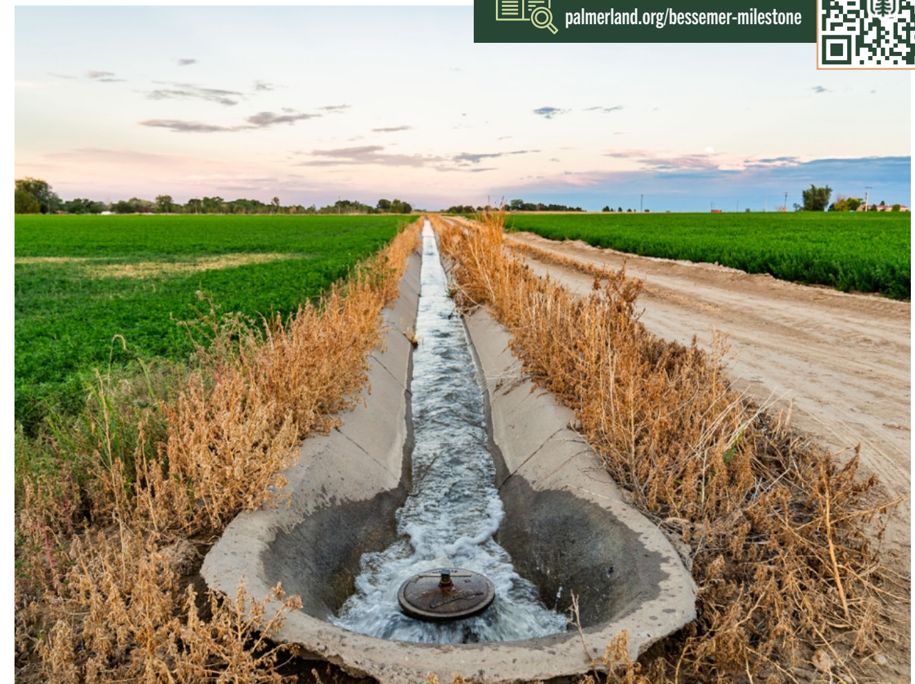
Bessemer farm irrigation system | Photo: Darrell Fisher and St. James Sporting Properties
