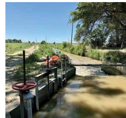
Las Animas headgates and irrigation flume | Photo: Dillon O'Hare
